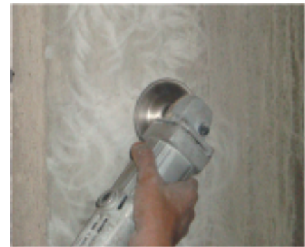
Concrete grinding
